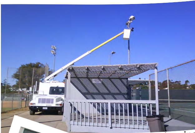
Finally cleaning the lights!
